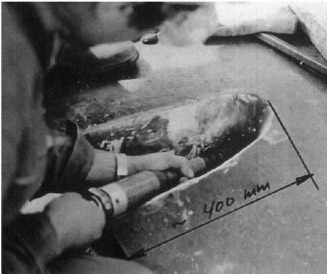
Fig. 1 Excavation and Weld Repair of Surface Flaw
